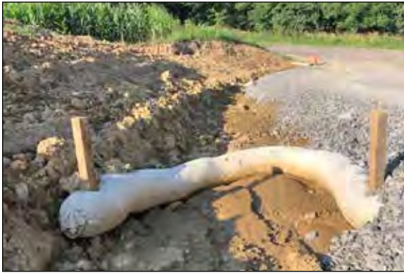
SiltSoxx NATURAL PLUS used as Check Dam.
